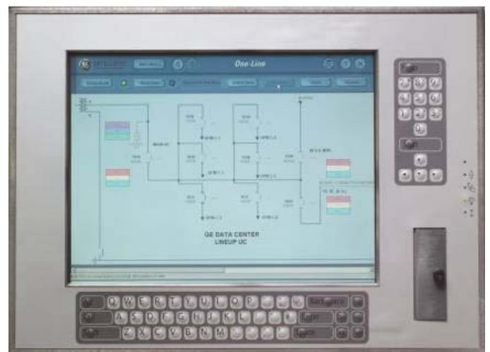
Figure 3: An example of an Entellisys switchgear touchscreen used for remote circuit breaker operation.
